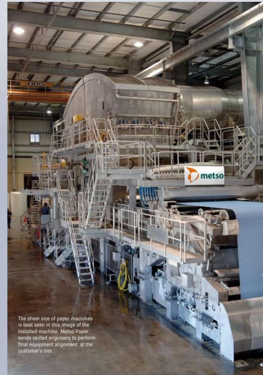
The sheer size of paper machines is best seen in this image of the installed machine. Metso Paper sends skilled engineers to perform final equipment alignment at the customer's site.
